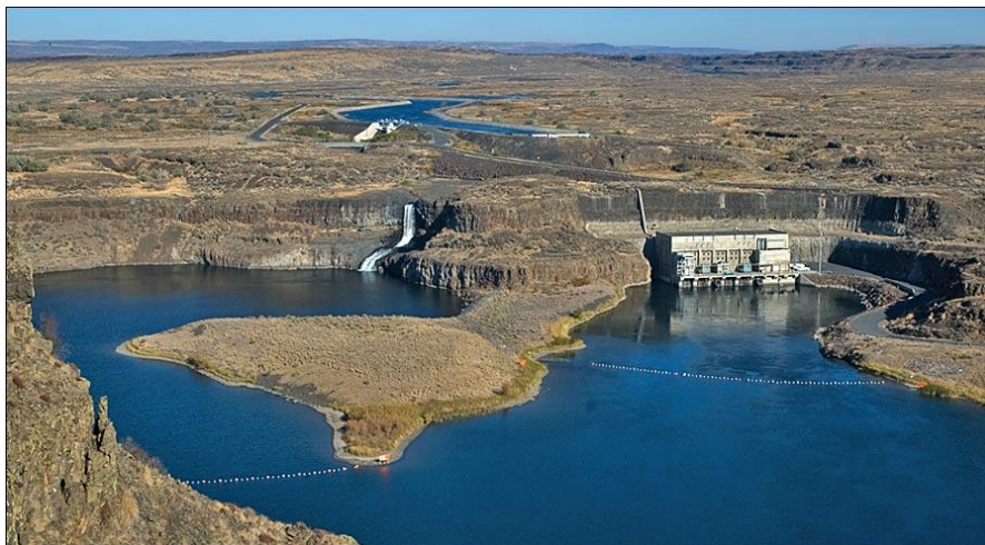
Figure 39: Part of Columbia Basin Project's Main Canal in upper-center background. On the left is Summer Falls (site of 1978's tragic triple drowning) pouring into Billy Clapp Lake. U.S. Bureau of Reclamation hydro-facility is on right. Photo clearly reveals ancient basalt lava flows of eastern Washington State. http://iceagefloods.blogspot.com/2008/10/billy-clapp-lake.html
