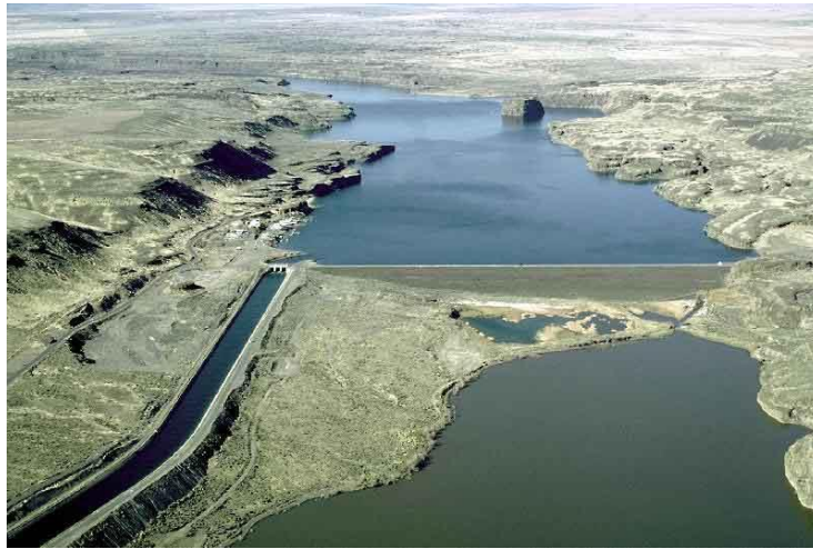
Figure 40: Pinto Dam at south end of Billy Clapp Lake with continuation of Main Canal on left front. Photo also shows the dryness and bleakness of the land.
