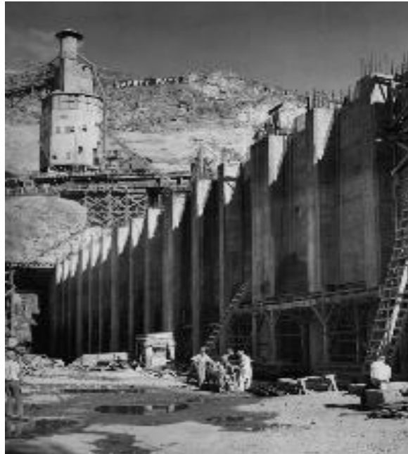
Figure 31: Construction of Grand Coulee Dam, 1935.
