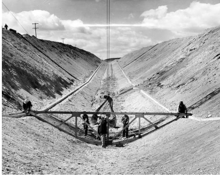
Figure 36: Construction of Columbia Basin Project's West Canal in 1947. http://www.trumanlibrary.org/photographs/displayimage.php?pointer=5825&people=&listid=4
