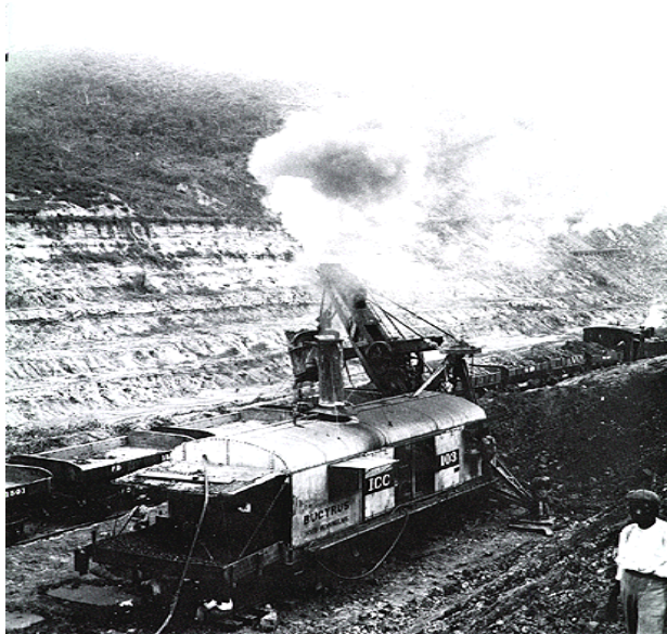
Figure 16: Steam shovel working in conjunction with railroad in Panama. http://www.latinamericanstudies.org/panama-canal3.htm
