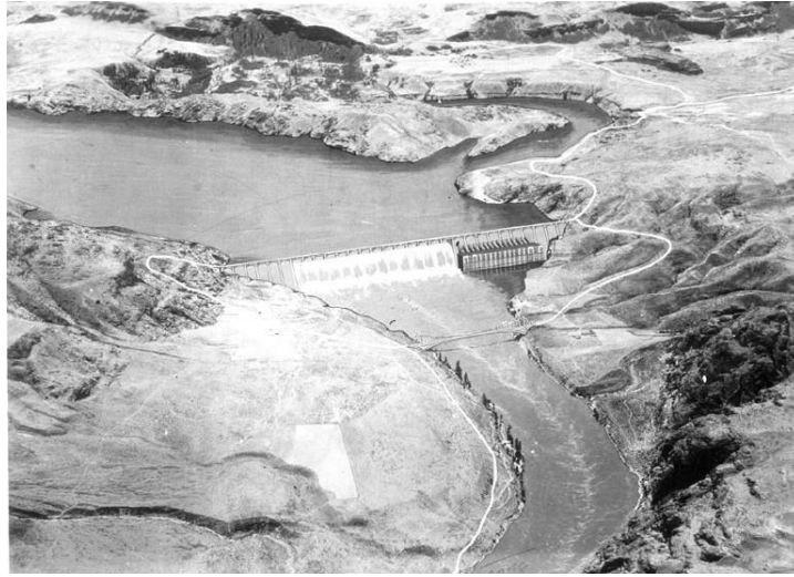
Figure 30: Early construction photo of Grand Coulee Dam, 1934.
